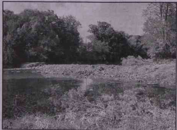
The concrete cap has been completely removed from the Nashville Dam.
