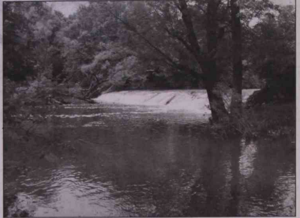
Local residents are invited to a hearing Tuesday, Aug. 25, to share views on the removal of the Nashville Dam.
