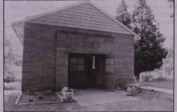
Erected in 1958, the Teen Smith Memorial Chapel includes a room that will seat 100 people and is being given a facelift by a group of community members. (Photo by Amy Jo Parish)
