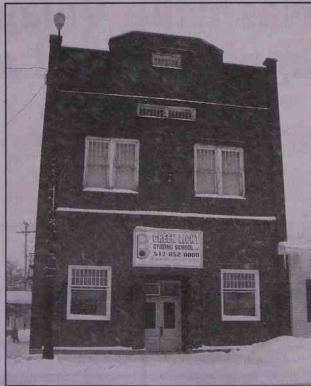
The Masonic Lodge in Nashville, owned by Dr. Michael Callton, will be the new home of The Revue.
