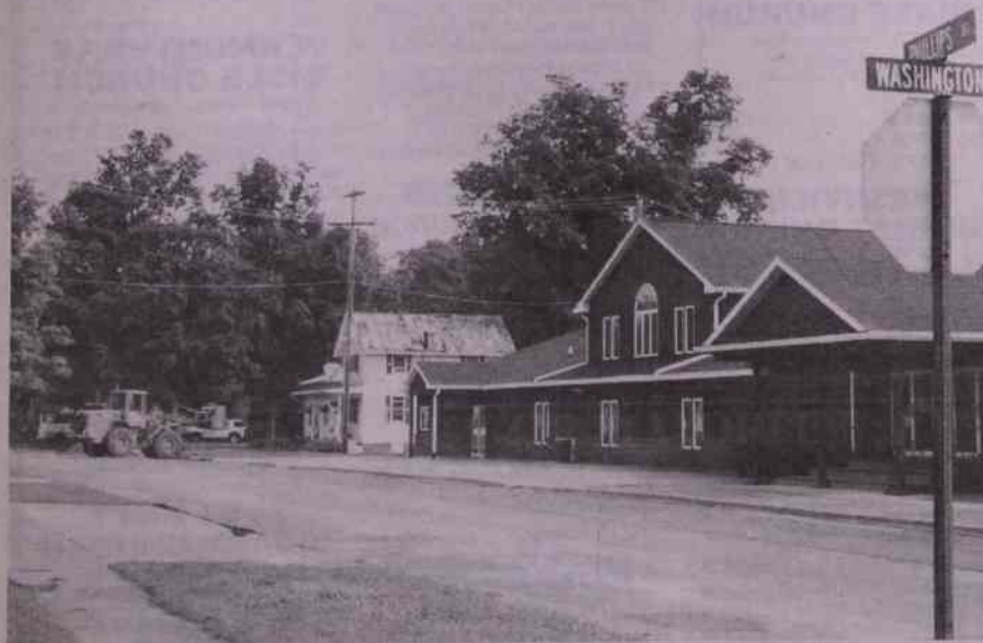
Work on the water main continues on Phillips Street.
