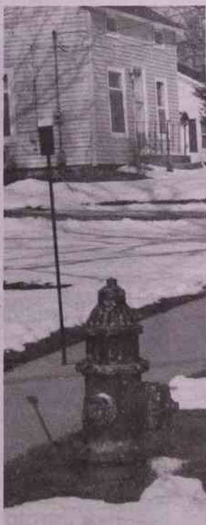
Fire hydrants in Vermontville now have flags so that even if there is heavy snowfall the hydrants can be easily located.
