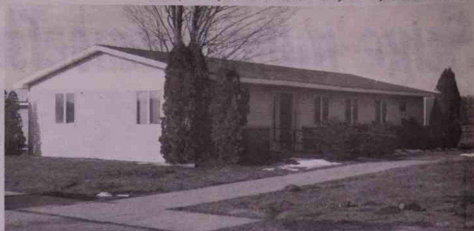
This is the administration office after it was resided.
