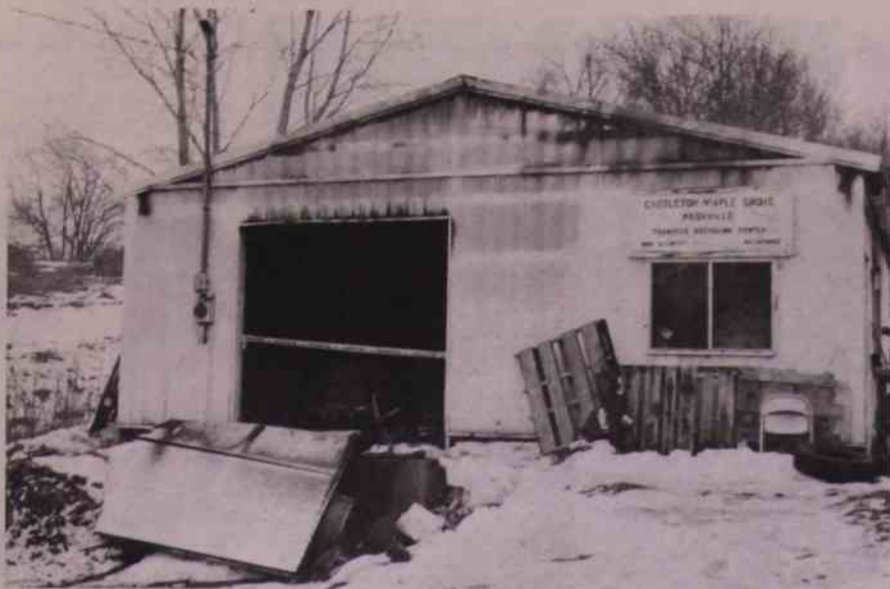
The Transfer Recycle Station sustained serious damage in a fire in February. Although the building was rebuilt, the station still faces economic troubles.
