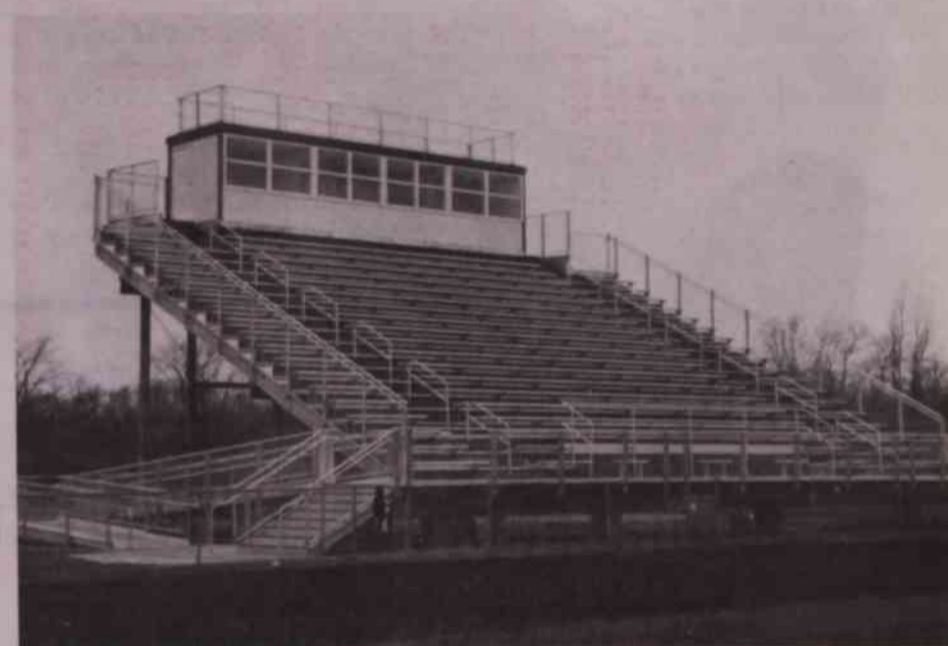
This year saw the first section of the new bleacher system up behind the high school. The bleacher system has handicapped access and a new press box.
